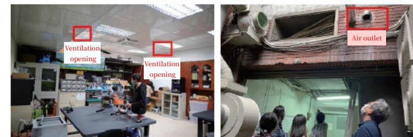
▲ Diagram (left) photograph of the basement (right)location of the air outlet opening of the thermal exchange device.
