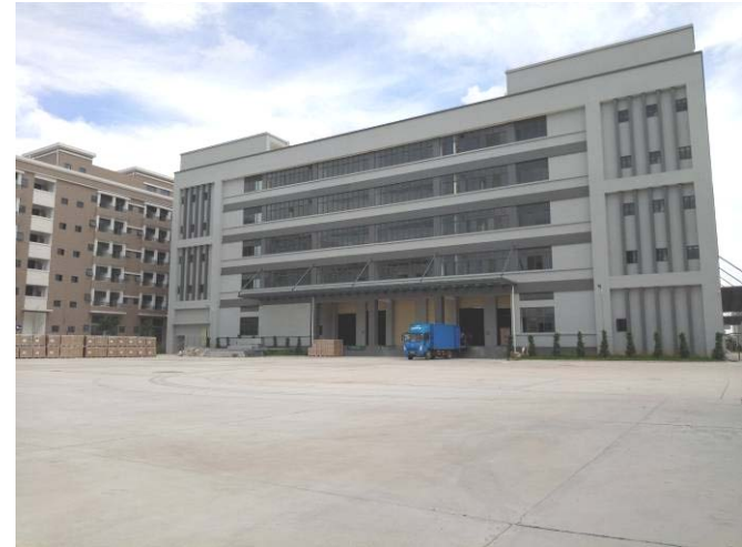
The building of warehouse
