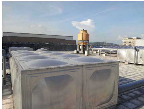
Environmental protection circulating water system
