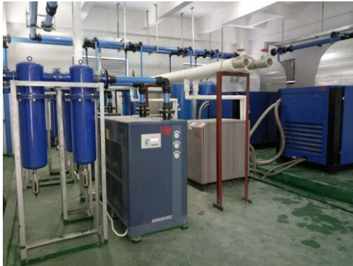
Intelligent environmental protection variable frequency air compressor system
