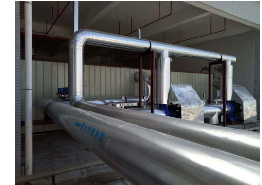
Intelligent environmental protection ice making system
