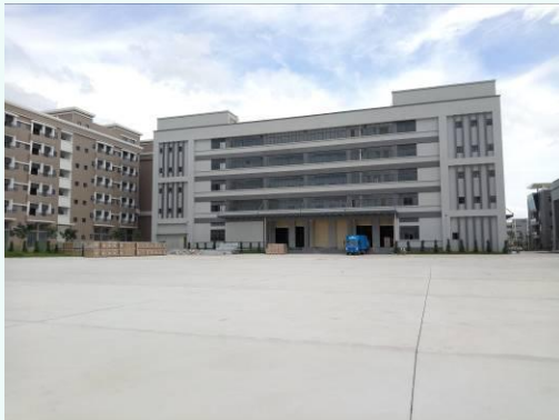
The square of shipping dock
