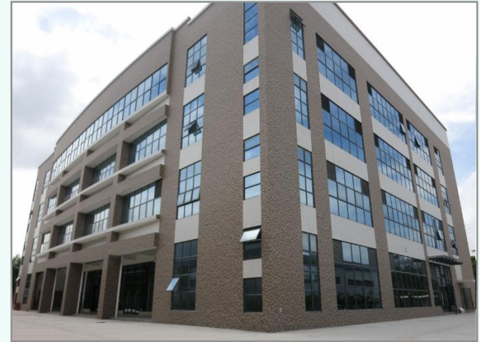
The building of leisure center
