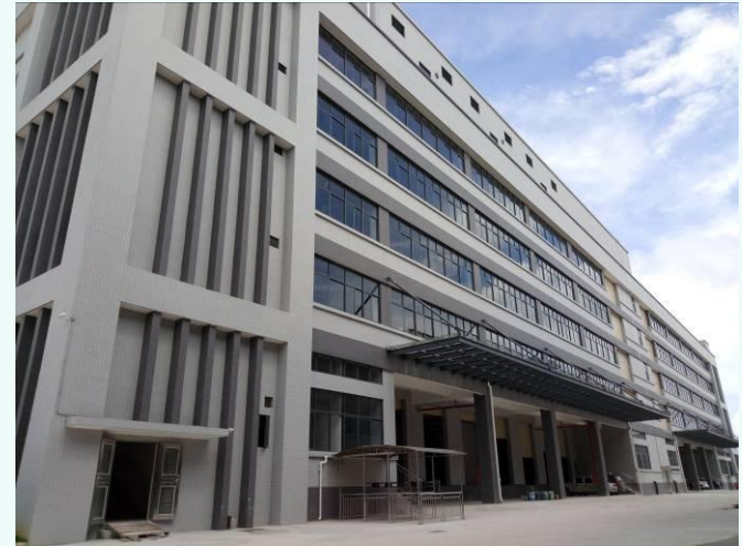
The building of AC production
